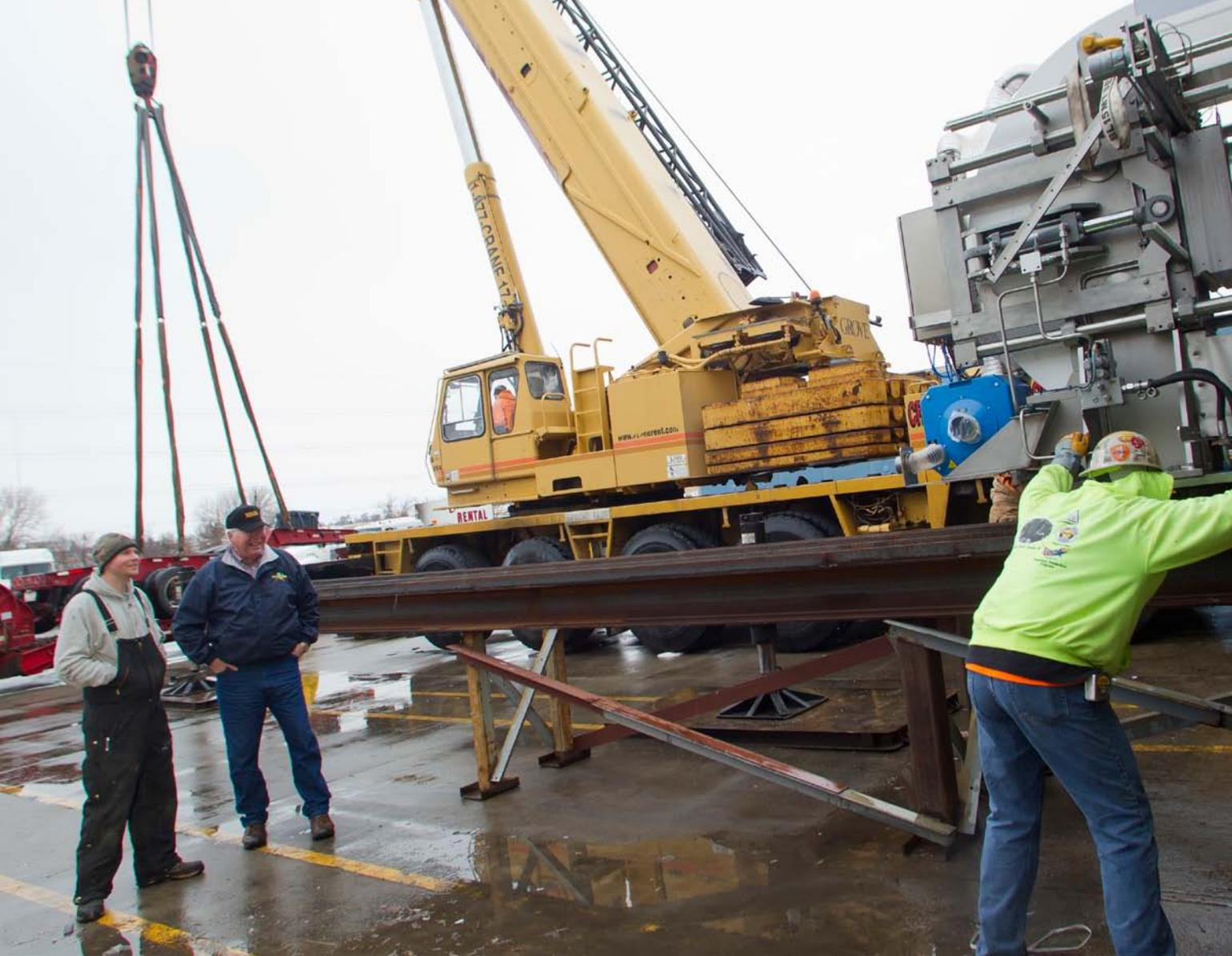
John Jacobson (second from left), owner/manager of UPC and Universal Cold Storage (UCS), observes the delivery of the company's fourth HPP machine, which was lifted by the large crane in the background onto rails to be rolled into the facility through the dock doors.
